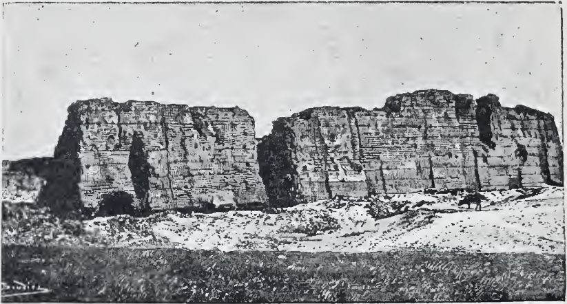
ONE OF THE FAÇADES OF THE FORTRESS OF KUBBÂN. 1
